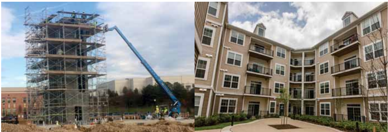
Oxford Square construction.
