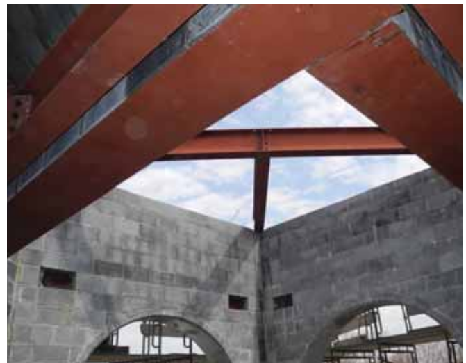
The Atholton HS renovation was recently completed.
