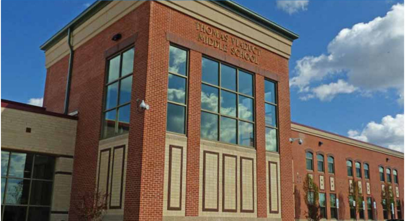
Thomas Viaduct ES opened in August of 2014
