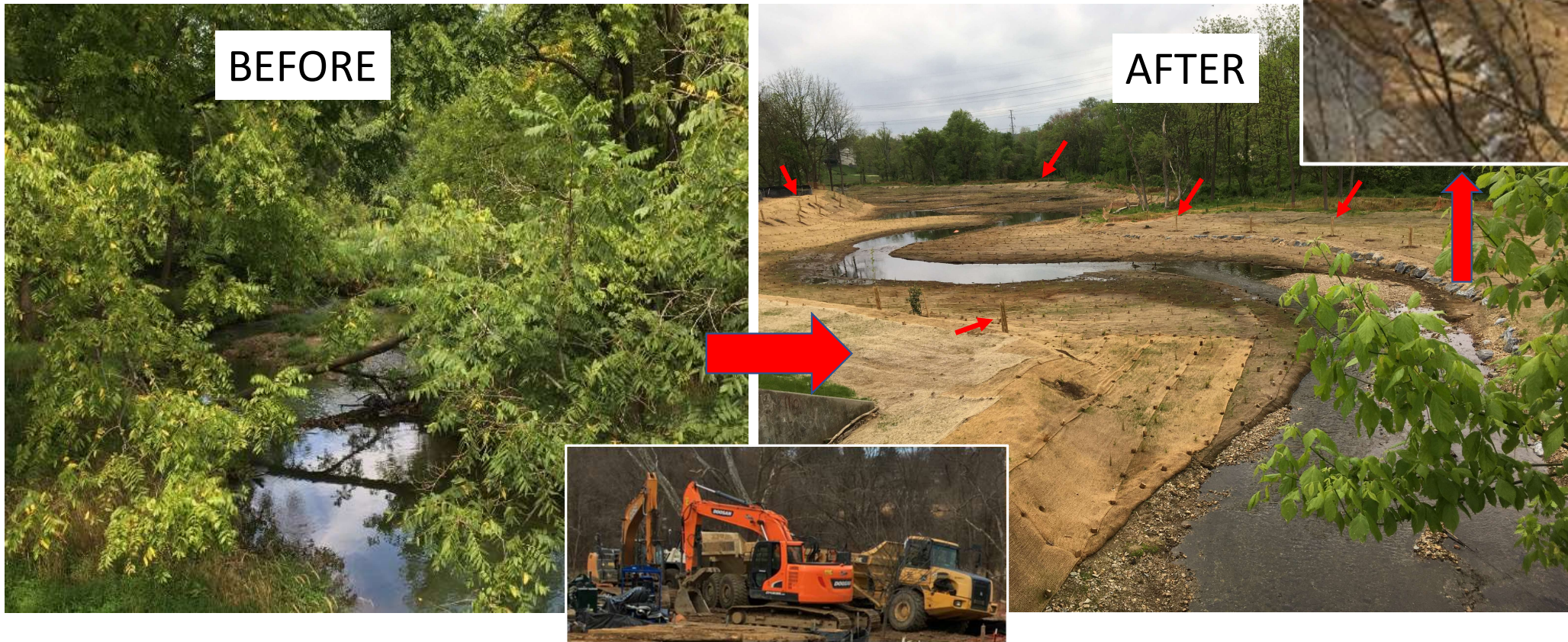
(Stream “restoration” in Blohm Park, Gaithersburg at Watkins Mill Rd. over Whetstone Run at the same location. Note the stream bank armor-plating on the right. (Left on 9/3/2020; right on 5/03/2021); by K.Bawer)
