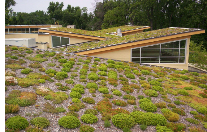
Green roof (by realfarmacy.com)
